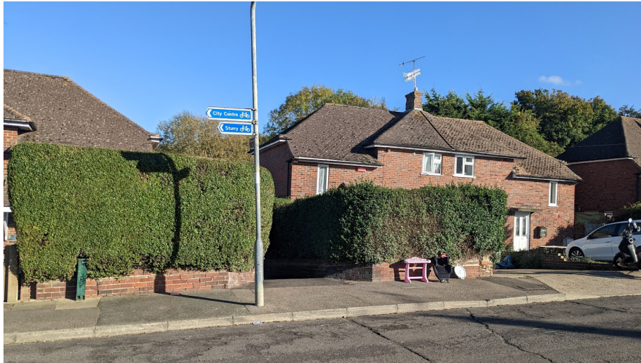
Image showing the lack of a dropped curb to footpath CC24.
